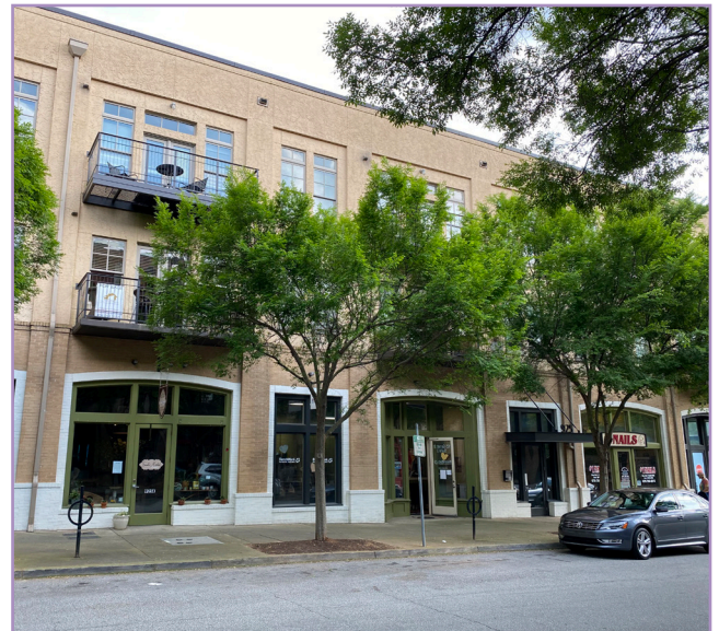
Figure 3: Apartments incorporated into a walkable retail development adds new housing options to the neighborhood
